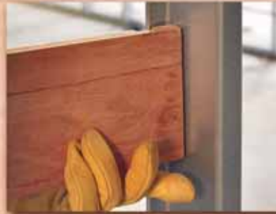
HINT: Start with the first full bay. Use Danback® Trimables for off-module bays.
