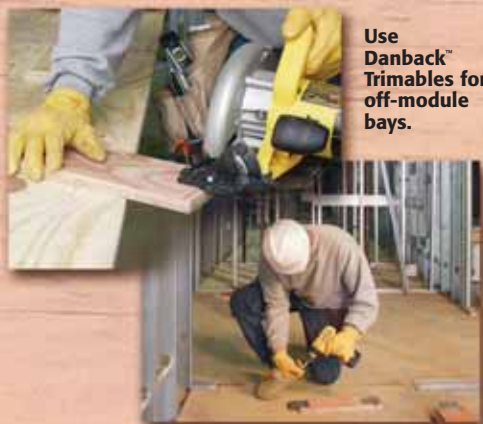
Cut to required length. Secure connector plate to the trimmed edge. Leave 1-1/4" extended over the trimmed edge. Fasten the plate to Danback using 3 small pan or wafer head screws.
