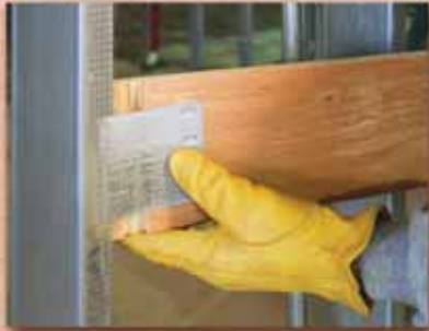
Snap "Starter Edge" into the open side of the stud flange.
