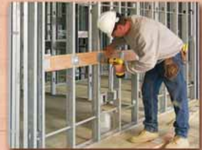
Secure each plate to the stud flange using 2 small pan or wafer head screws.
